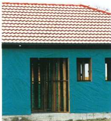
"Wrapped and sealed in a barrier."
